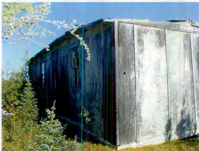
Photo 13. Aerial view of Site 321A before (September 8, 2000) and after clean-up (September 11, 2000). View behind building where the foundation has collapsed.
