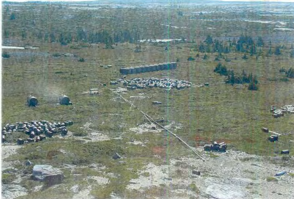
Photo 11. View of Site 403A before clean-up (September 12, 2000). Compare with diagram in Appendix 3.
