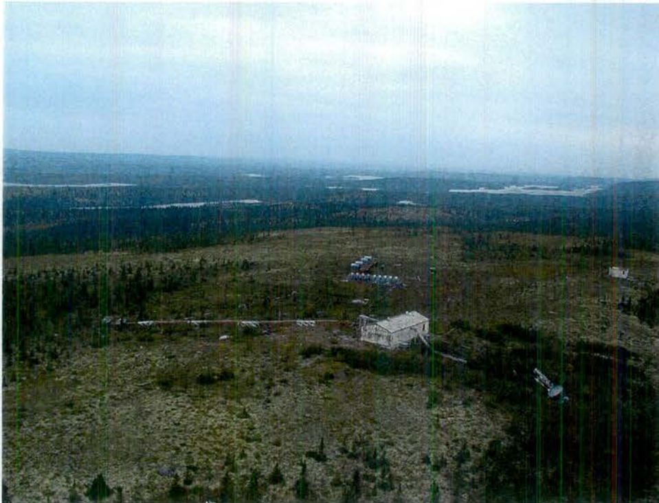
Photo 1. Typical detection site located on the top of a hill with a main building, a survival shelter, fuel tanks, barrels and two tall antennas.
