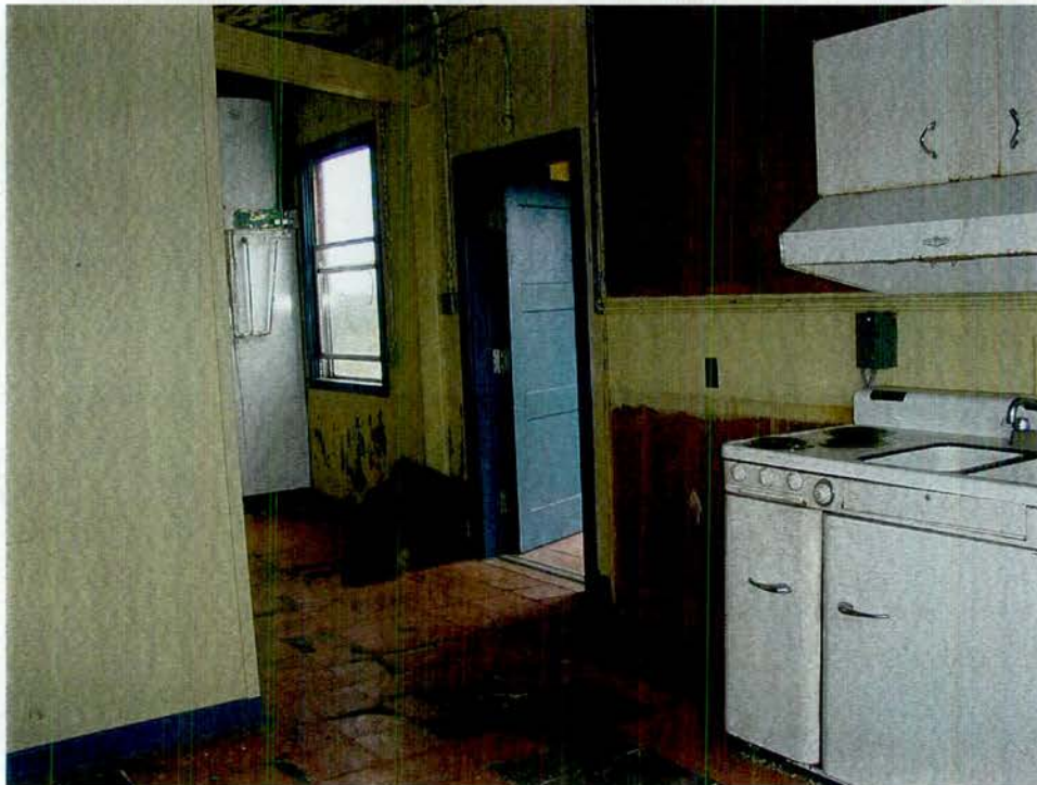
Photo 8. Equipment room and kitchen at Site 330, after clean-up (September 6, 2000).
